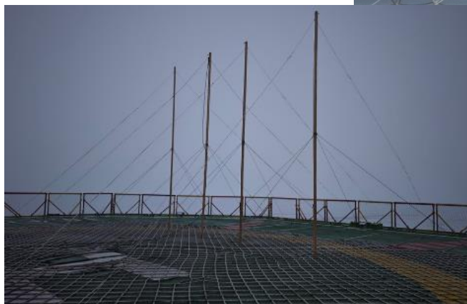
18МГц – 3 el Yagi 17m 3el Yagi 9m up Gain = 11,5dBi
