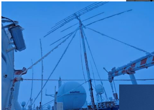
18МГц – 3 el Yagi 17m 3el Yagi 9m up Gain = 11,5dBi
